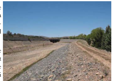
Lynx Creek Levee protecting Orchard Ranch RV Park
