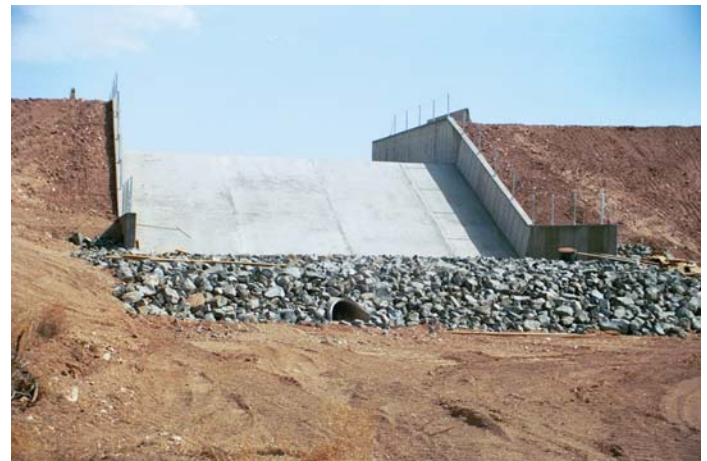
The Wineglass Dam spillway project, during construction, above, and at completion, below, was designed as a result of the State's determination to remove the dam from the unsafe dams list. By adding the spillway, the dam was able to remain in place and continue to provide flood protection to the properties below.
