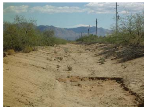
The Paso del Sol Subdivision in Congress benefitted from a channel that the District designed and built to protect properties in the floodplain.
