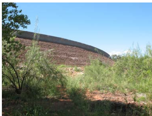
Dry Creek Levee protecting Sedona Shadows
