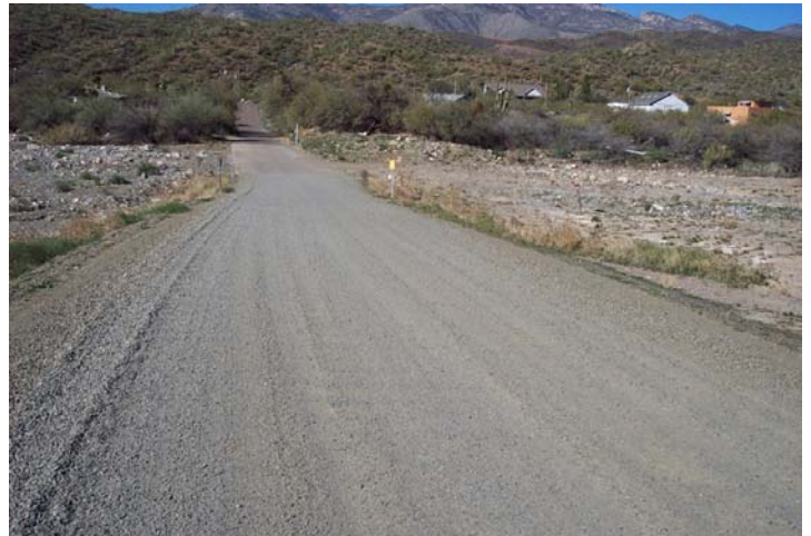
Maren Drive across Black Canyon with a temporary road crossing today, above. Squaw Valley Road across the Agua Fria River with a new low water crossing, today, below.
