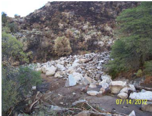
Debris flows fill the sediment traps upstream of Crown King Road, above. Boulders are washed into the roadway after the stabilizing vegetation is burned away, below.
