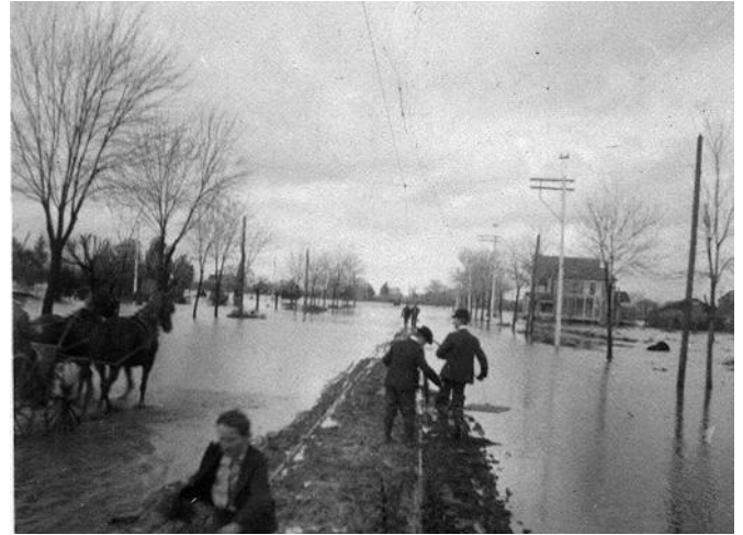
The railroad is covered in water early last century.
