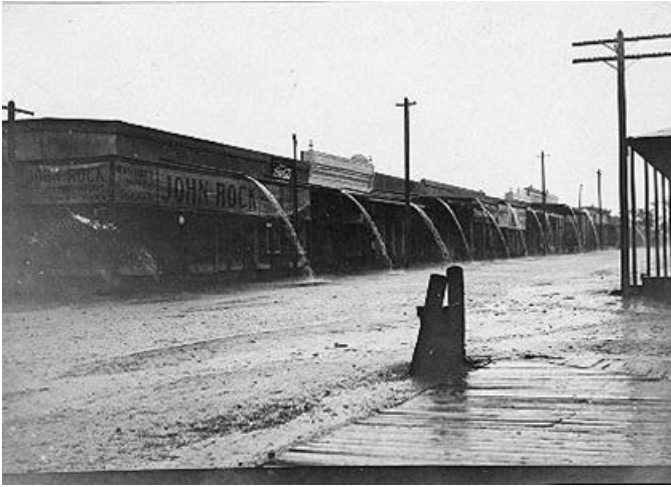
Roof drains rain down on the street.
