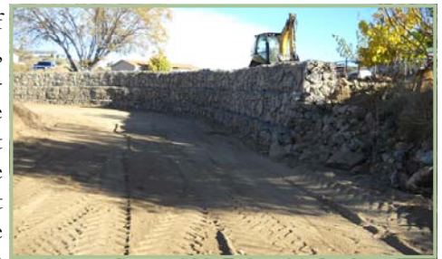
Portions of South Rocky Boy Wash were lined with gabion baskets.
