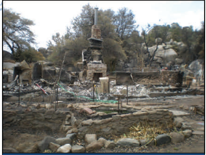
Destroyed residence in Yarnell, AZ
