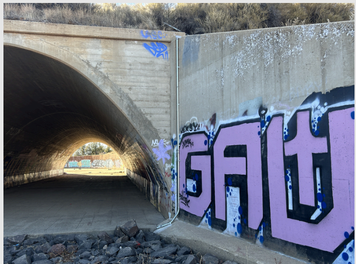
This photo shows the channel downstream and the conduit and sensor for measuring stage (water level)
