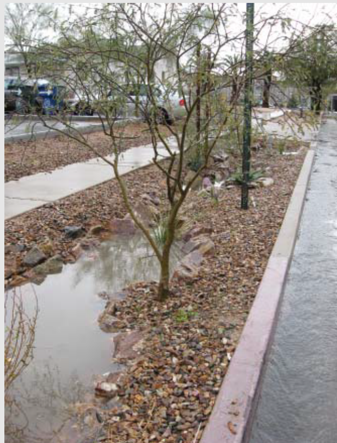
Below: A newly completed curb cut with rock-lined basin in action in a City of Tucson right of way.
